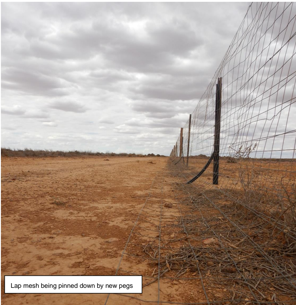
Rebuild floodgate (Marree)
