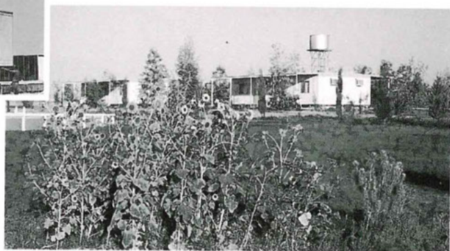
A view across the attractively established grounds at the head-quarters of the Ain Kawah project. Extensive lawns, Eucalypt plantations, a swimming pool and flower beds helped make the South Australian project a pleasant site envied by other expatriates in Iraq.
