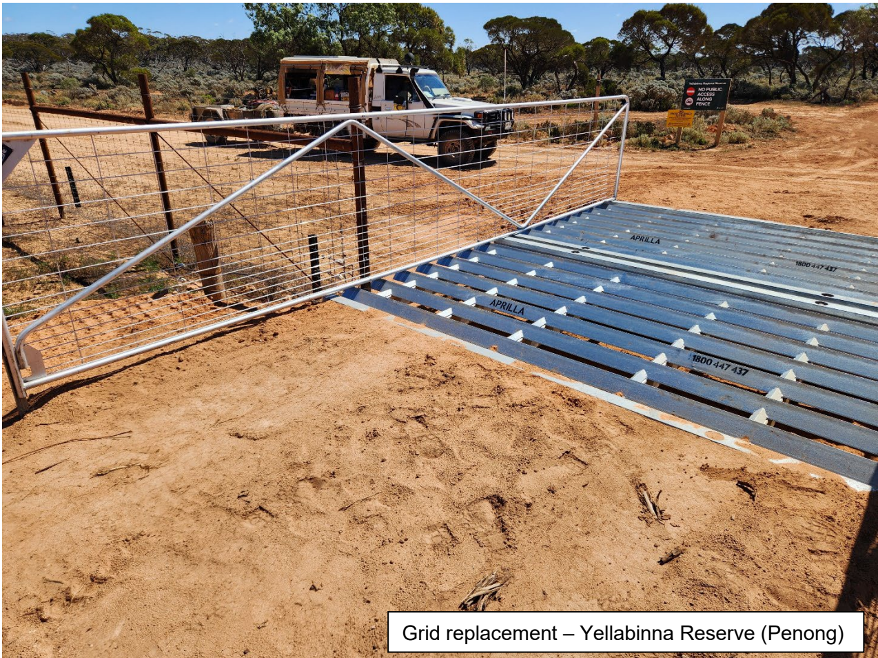
Grid replacement – Yellabinna Reserve (Penong)
