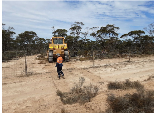
Image 6 - Telstra working through the new fence
