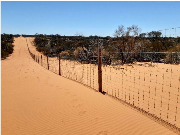
Image 7 - Fence heightening at Lake Everard due to sand drift
