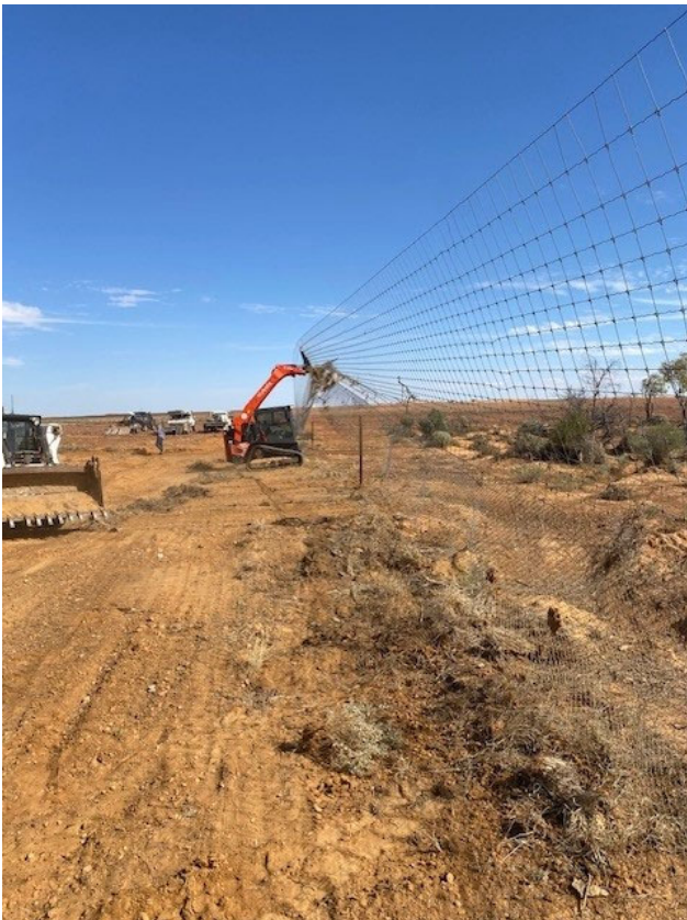
Image 3 - Flood repairs at Mundowdna
