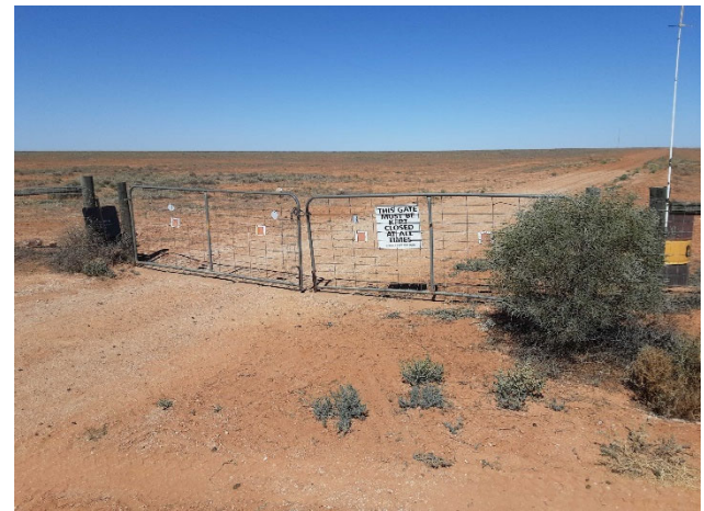
Image 4 - Double gates on the pipeline road
