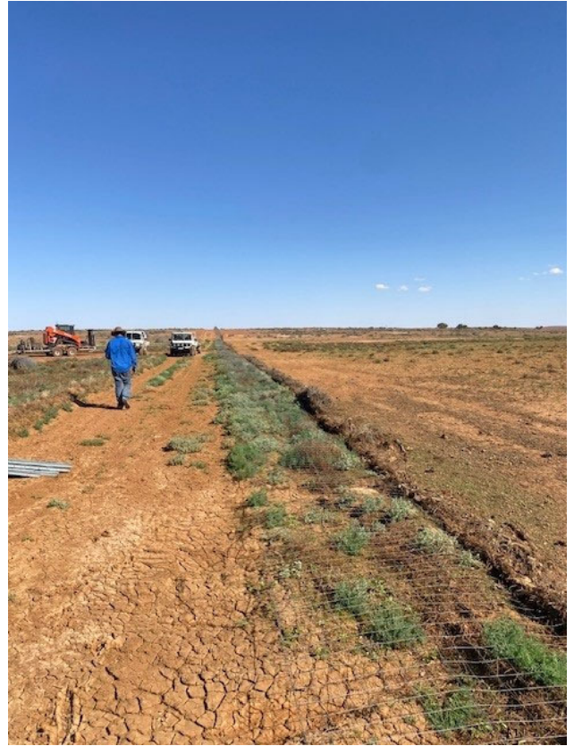
Image 2 - Flood repairs at Mundowdna
