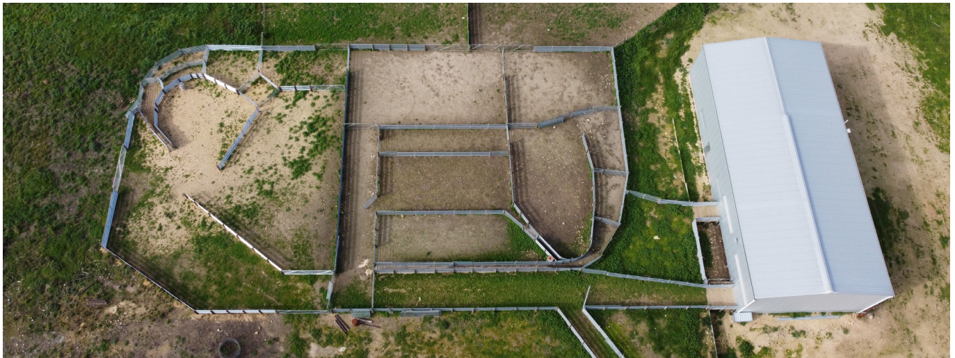
Figure 3: Layout of yards at Rangefield, showing satellite yard specifically designed to accommodate auto-drafter and contractors' equipment
