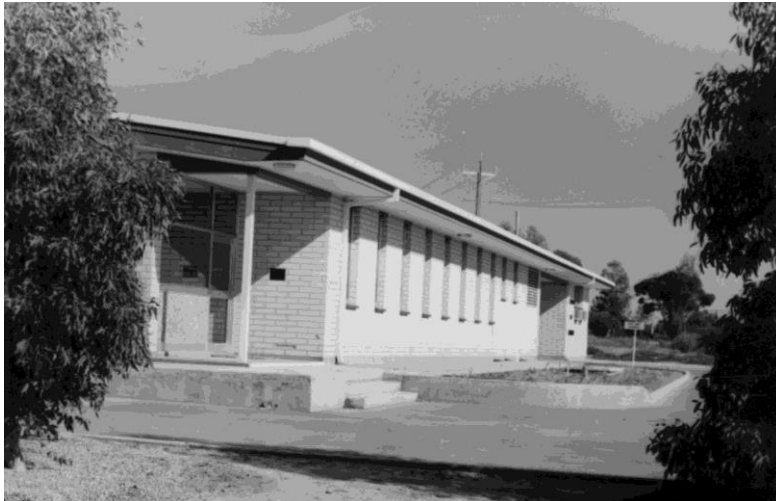
Initial office and laboratory complex, Loxton Research Centre, 1973.
