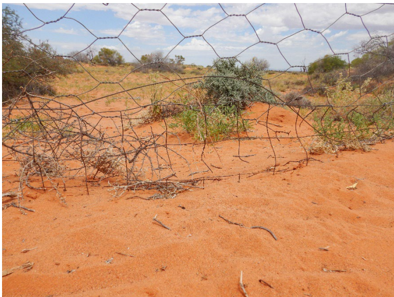
Rust damage to foot netting/strainer wire – Wertaloona
