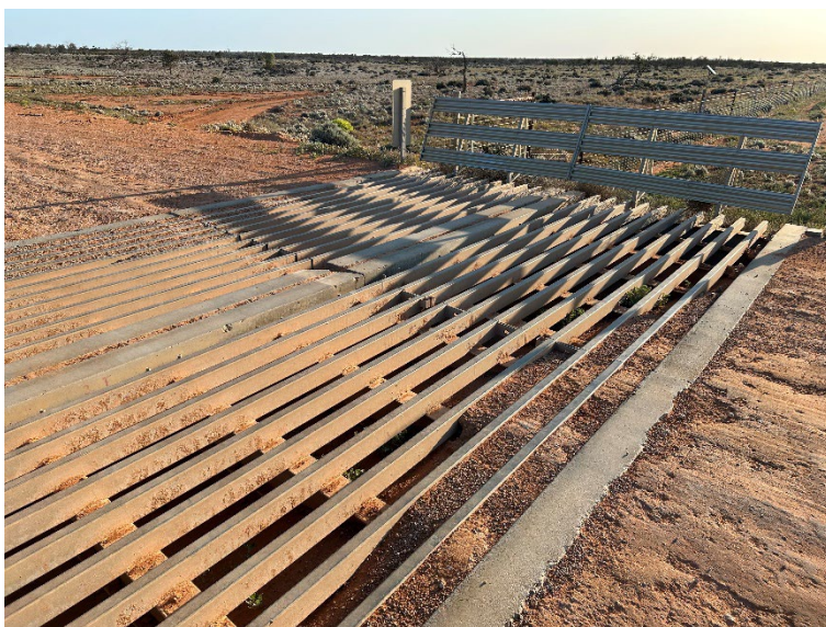
Tea Tree Road Grid – North side
