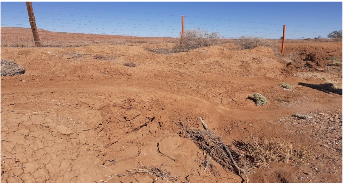
Minor Track repair - Before
