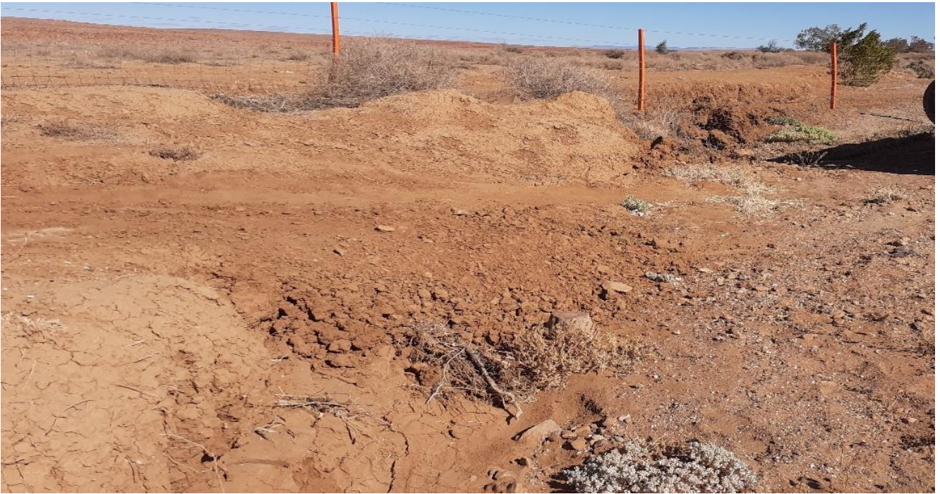
Minor Track repair – After
