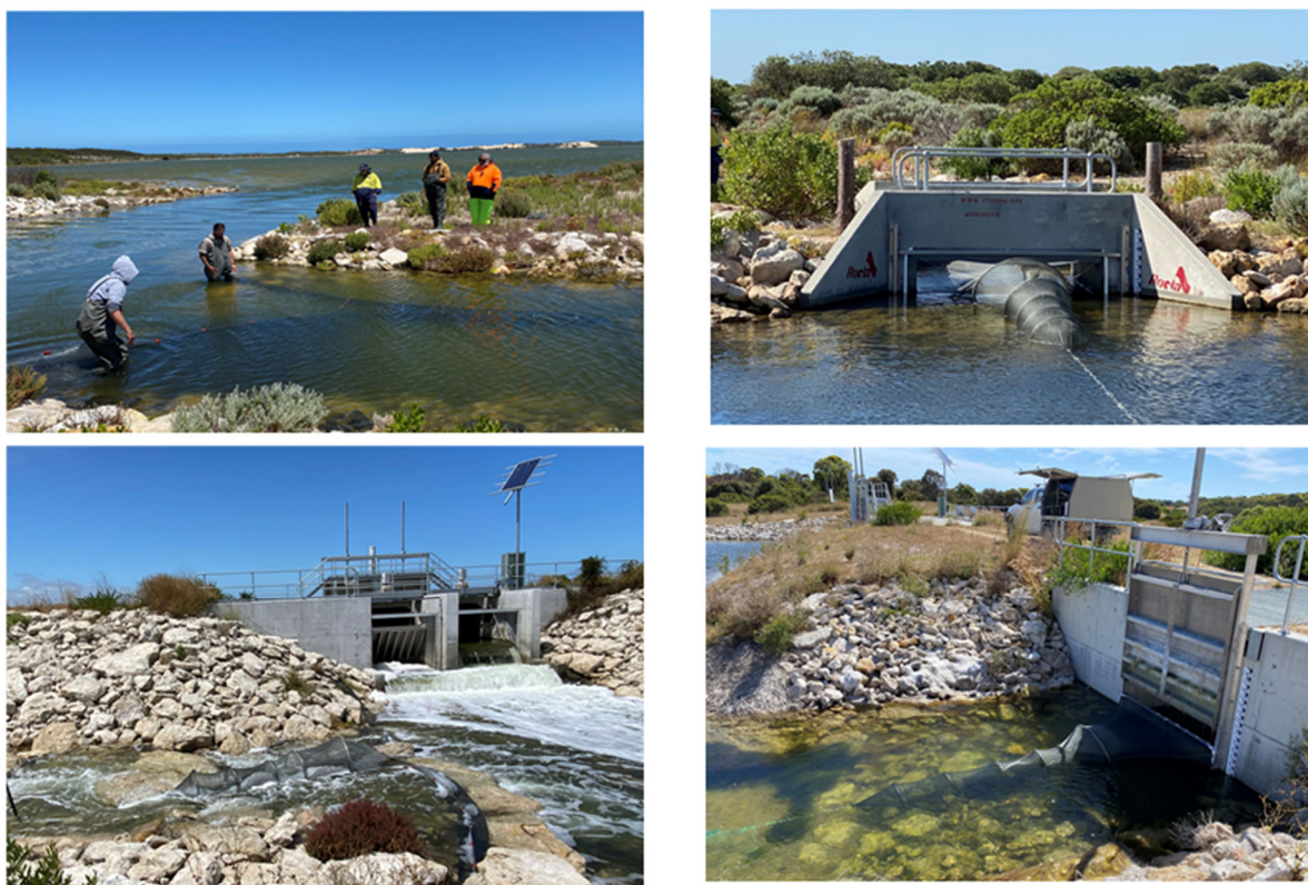
Figure 2.5. Fish trapping at the Salt Creek rock-ramp fishway entrance (top left) and exit (top right) and the Morella rock-ramp fishway entrance (bottom left) and exit (bottom right).
