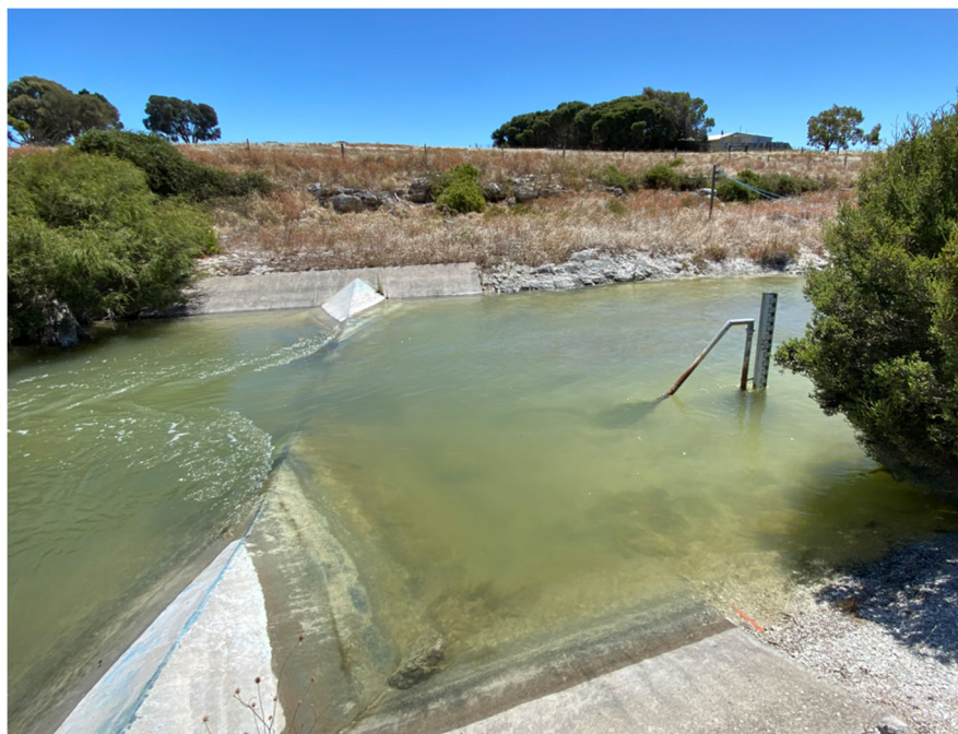
Figure 3.2. Crump Weir gauging station for water levels within Salt Creek.
