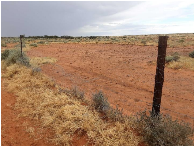
Fence damage caused by cattle activity
