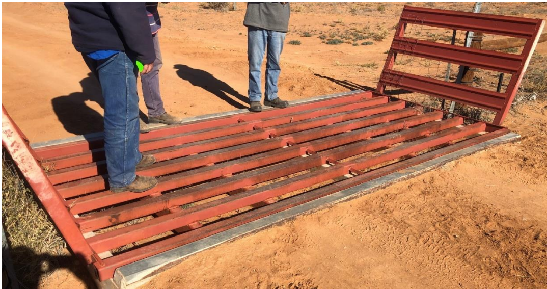
The Balcanoona grid which the Board plans to replace
