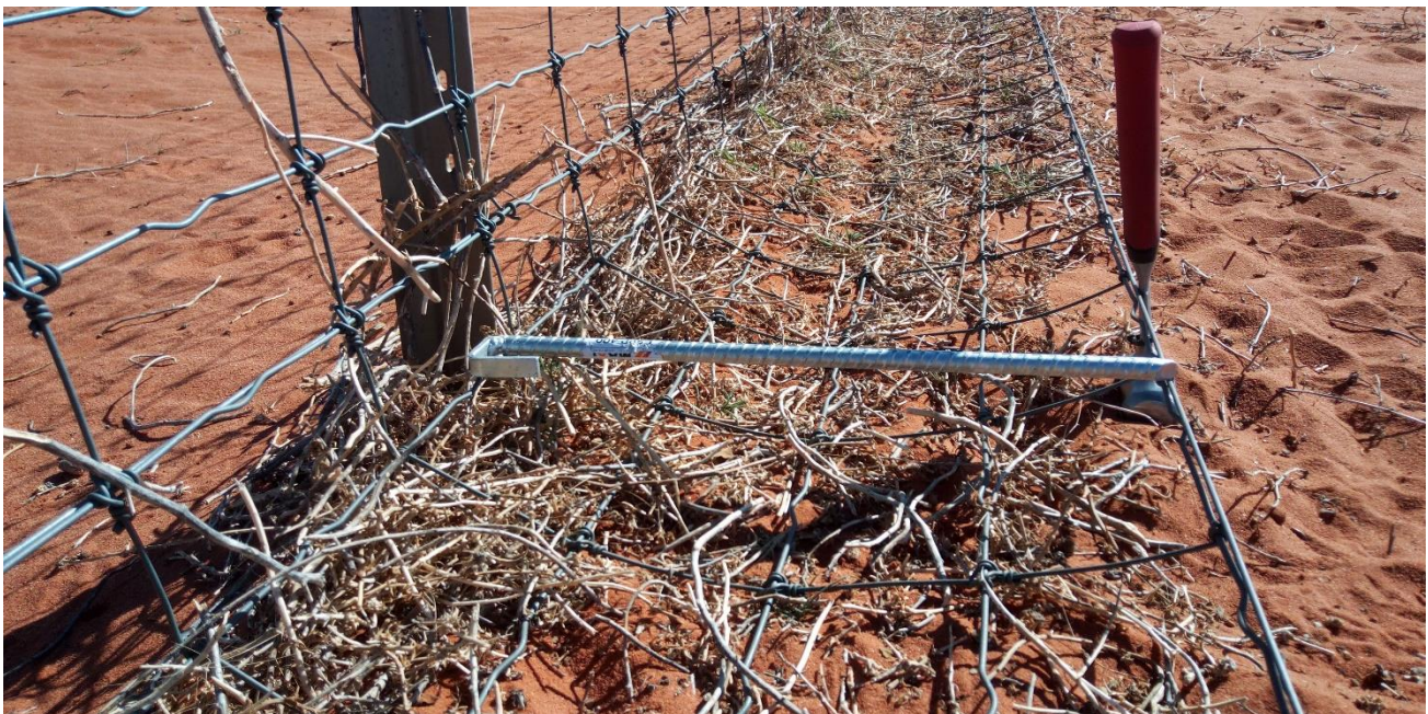
Reo-rod peg before fitting showing lap lift
