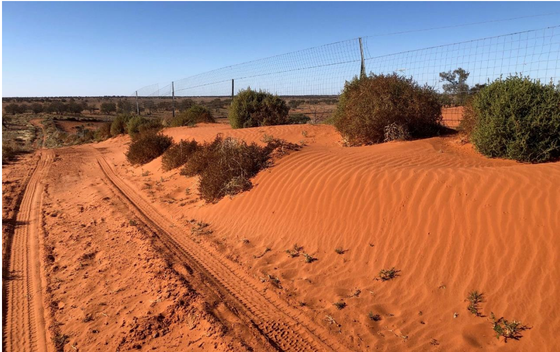
One of several sections requiring urgent topping due to sand dune height increase
