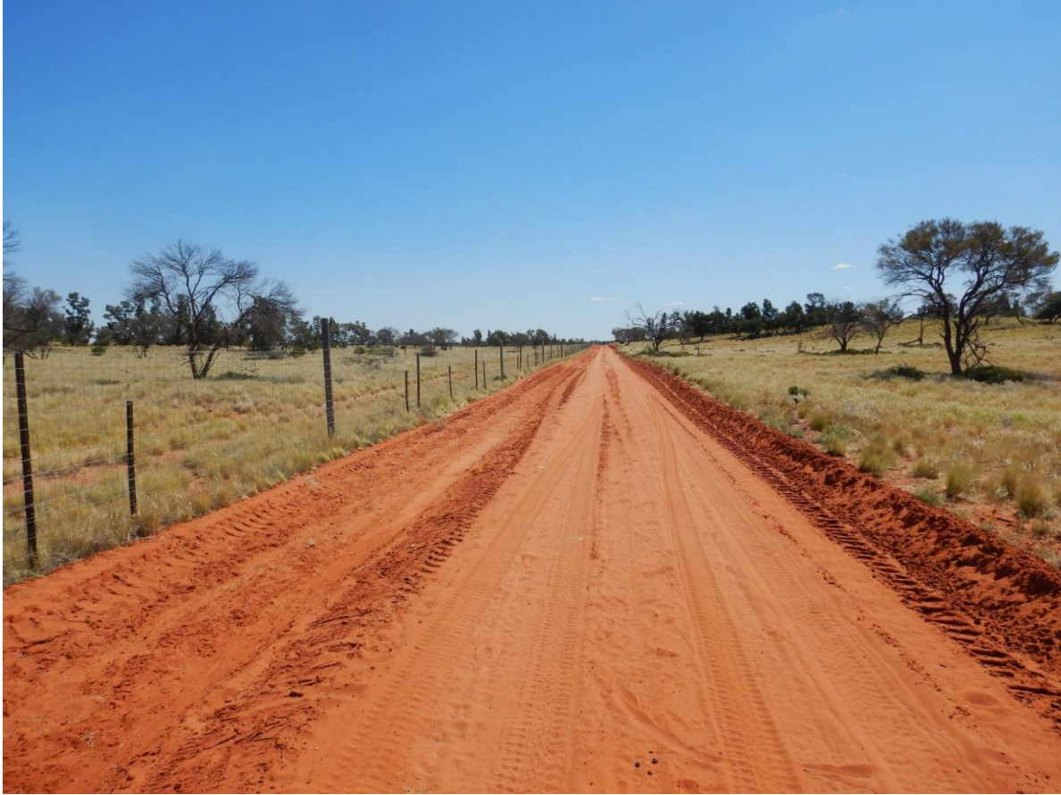
Completed earthworks - Parakyliia fence (Central LDFB)
