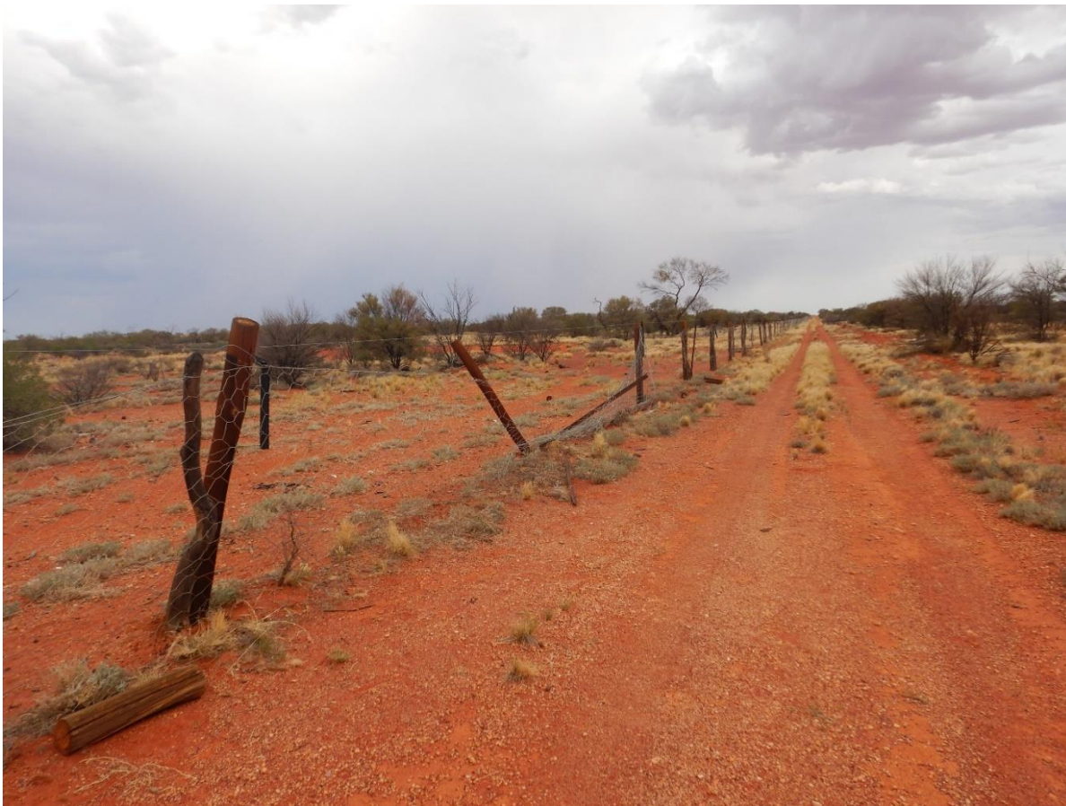
Camel damage sustained to fence – Mabel Creek (Central LDFB)
