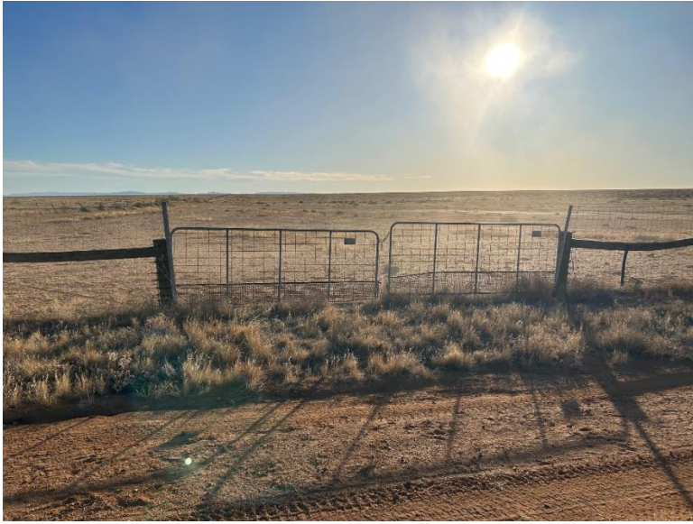
Moolawatana gate at 1200mm – Gate to be topped with netting or replaced
