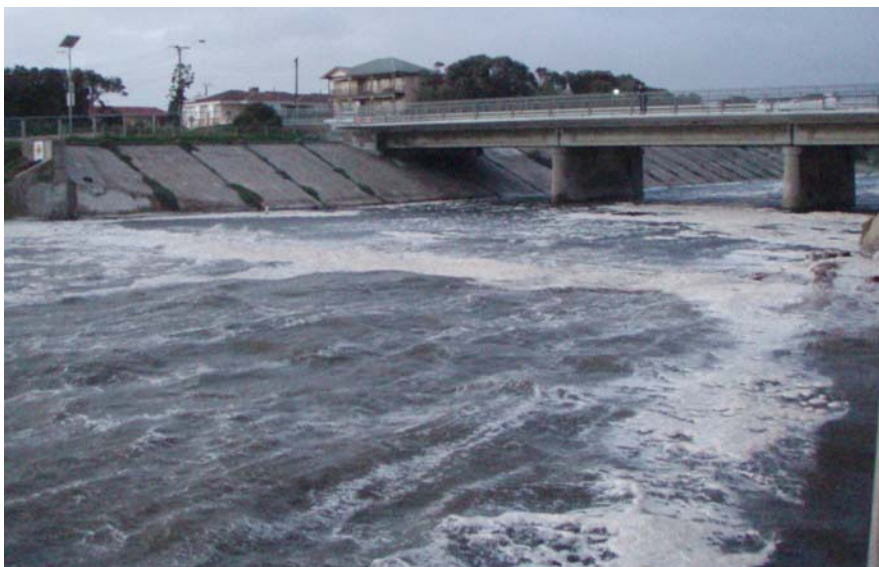
Figure 14. Seawater intrusion under high tidal and storm surge conditions in 2008 forcing Breakout Creek to flow backwards temporarily. This scenario provides opportunity for upstream migration from the sea without reliance on the fishway.
