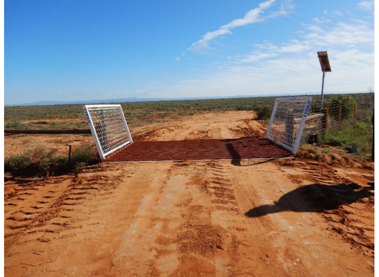
Balcanoona grid replacement
